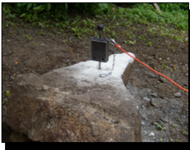
Figure 5—The BMS Micro-Blaster is ready to fire.
