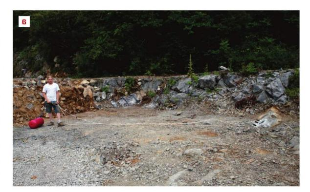
6. With the Micro-Blaster, debris rarely travels more than half the length of the air hoses, so blasting is much safer than with traditional charges. In close quarters, a scrap of carpet is enough to contain blast debris.
