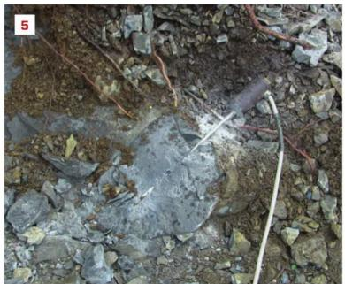
with each charge. It's important to drill the hole to the proper depth—a single charge requires a 10-inch-deep hole. If the hole is too deep, the firing pin won't be able to engage the cartridge.
